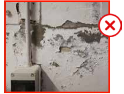
Fig. 5 | Pareti scrostate e rovinate
