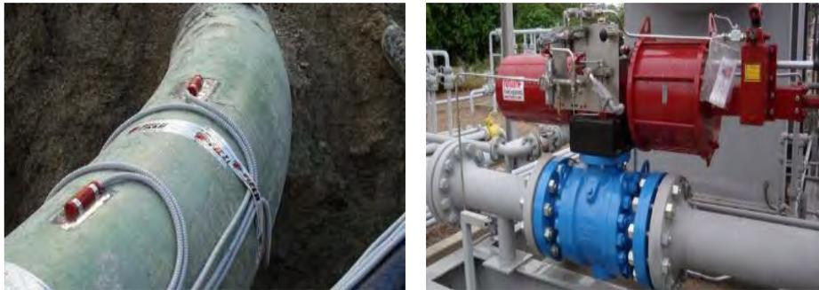
Figura 2. Strain Gauges e Shutdown valves
