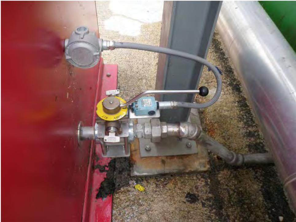
Figura 7. Valvola di intercetto CO<sub>2</sub>
