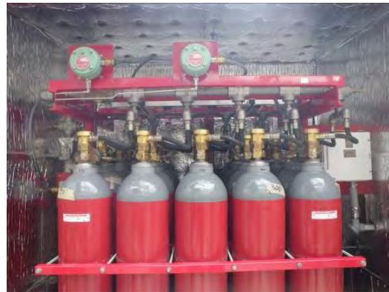
Figura 4. Bombole CO<sub>2</sub>
